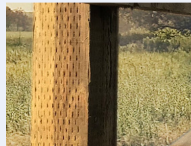
Mechanical incising of the surface is now used widely to help achieve the desired penetration of preservative.
