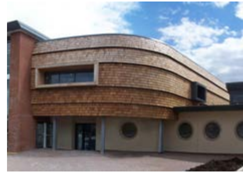
Primary School, Swansea
