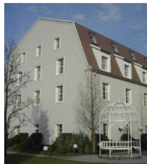
Bell Rock Hotel, Europa-Park External timber cladding prior to coating FR Specification: WPA Type INT2 (Humidity resistant)
