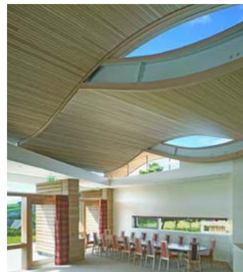
Robin House Hospice, Leeds Interior and exterior timber cladding FR Specification: WPA Type INT2 (humidity resistant for internal)
